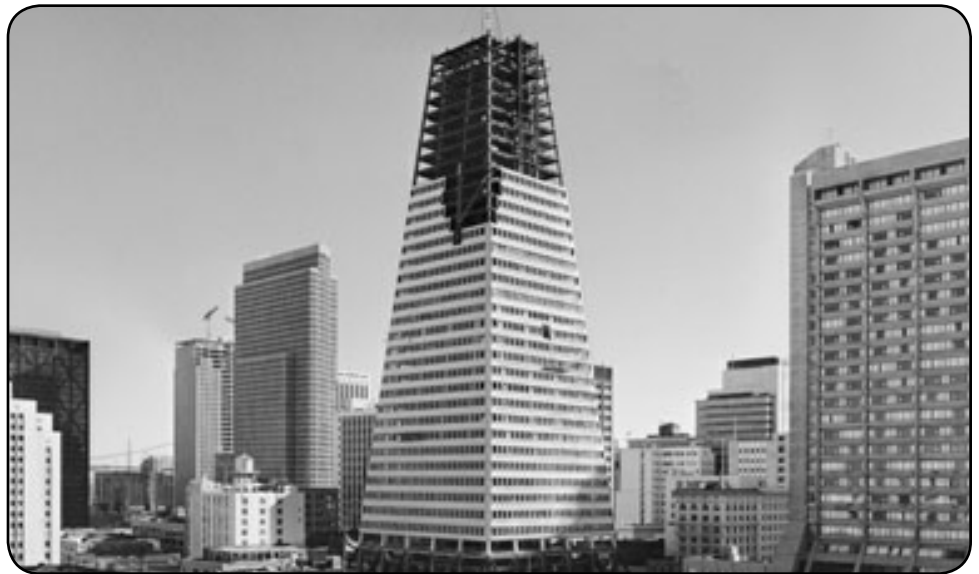
Construction began in 1969 and was completed in 1972.
