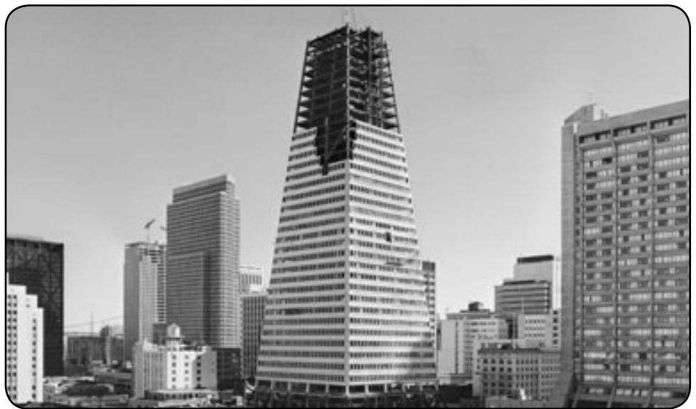
Construction began in 1969 and was completed in 1972.
